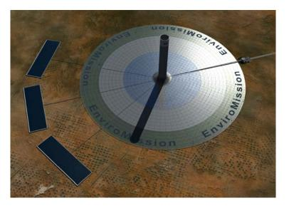
Solar Towers are designed to cause a constant flow of solar heated air to drive turbines to generate electricity based on solar thermal updraft principals. Air beneath a low circular translucent roof (collector) open at the periphery is heated by solar radiation (greenhouse effect) and naturally rises to the highest point – the base of the tower located at the center of the collector (the collector has a gradual slope toward the center).
