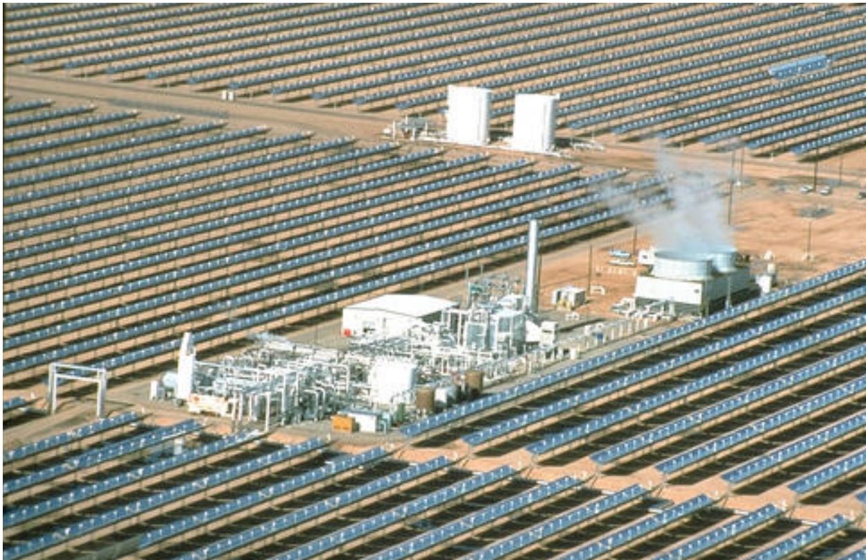
21 22 FIGURE 5.12-8 Power Plant at Commercial-Scale Parabolic Trough Facility (Credit: Sandia 23 National Laboratories; Source: NREL 2009a) 24 25
