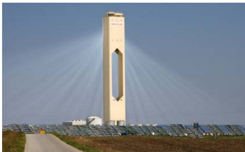
31 32 FIGURE 5.12-11 Solucar (Spain) Solar Power Tower and 33 Heliostats, with Visible Dust Particle “Tent” (Source: Flickr 2009)
