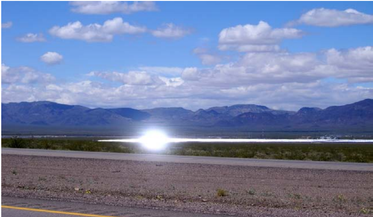
25 26 FIGURE 5.12-6 Glare from Parabolic Trough Facility at Distance of 2.0 mi (3.2 km) 27 (Credit: Argonne National Laboratory)
