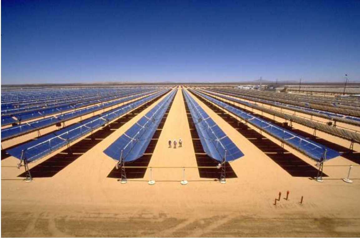
FIGURE 5.12-2 Trough Collectors for the Parabolic Trough Facility, Kramer Junction, California (in addition to CSP, the facility also includes a natural gas-fired turbine located in the facility's power block; see background right) (Source: Hosoya et al. 2008)
