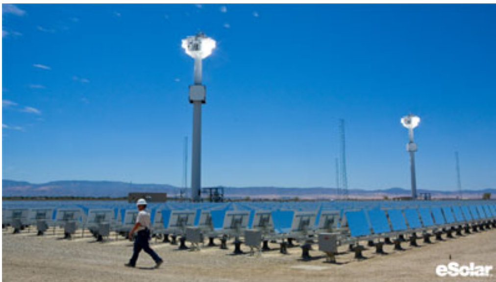
29 30 FIGURE 5.12-12 Solar Power Towers and Heliostats at the eSolar Sierra 31 Suntower Facility in Lancaster, California (Source: eSolar 2010)
