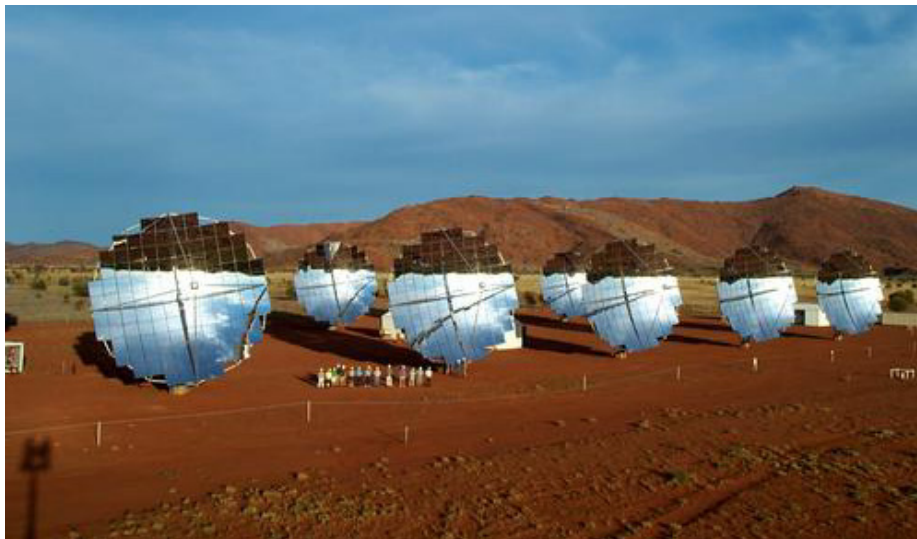
30 31 FIGURE 5.12-13 20-kW Solar Dish Engine Units in Alice Springs, 32 Australia (Credit: R. McConnell; Source: NREL 2009c)
