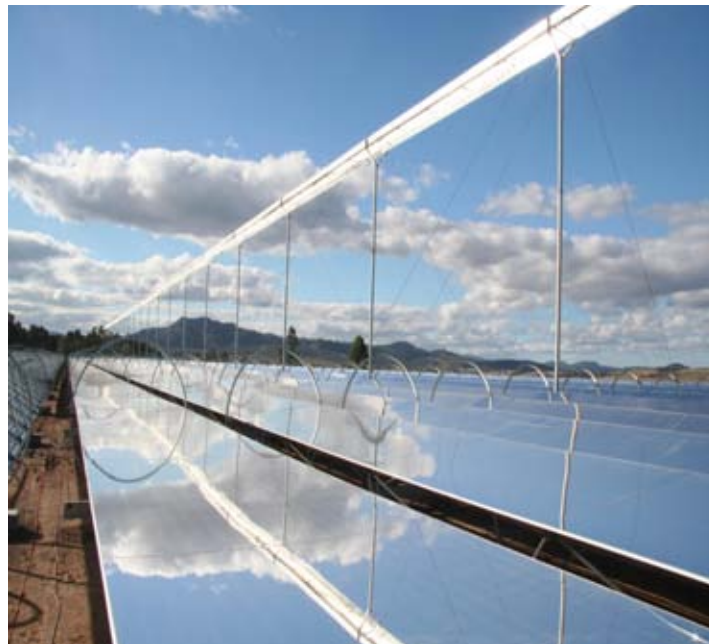
29 30 FIGURE 5.12-9 Commercial CLFR Solar Array 31 (Source: DOE 2009)
