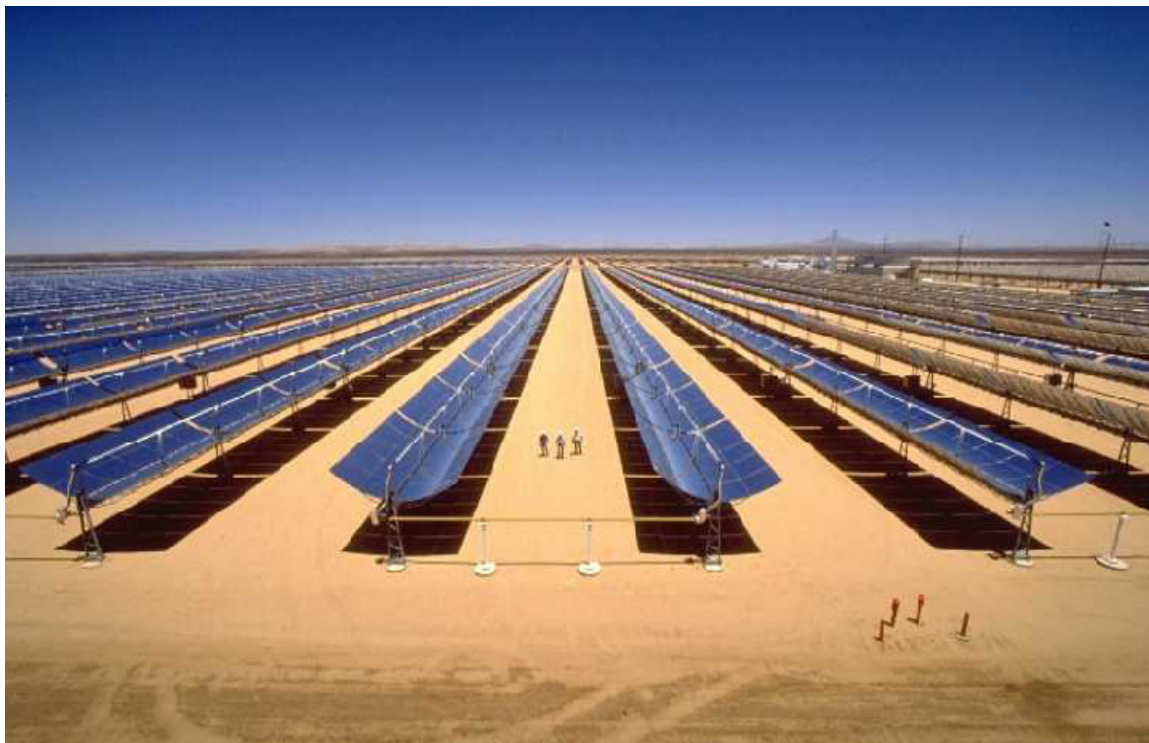
24 25 FIGURE 3.1-1 Solar Field for the Florida Power and Light Parabolic Trough Facility 26 Known as SEGS VI, Kramer Junction, California (Source: Hosoya et al. 2008)
