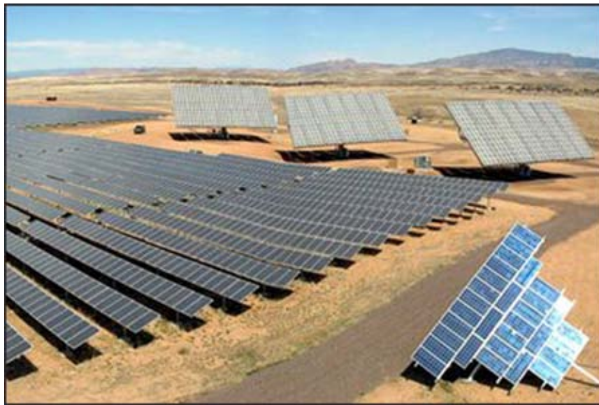
23 24 FIGURE 3.1-4 Utility-Scale Flat-Plate PV System at the Prescott, 25 Arizona, Airport Operated by Arizona Public Service Company 26 (This system incorporates flat-plate non-concentrating solar 27 panels [foreground] and concentrating flat-plate solar panels 28 [background].) (Credit: Arizona Public Service; 29 Source: NREL 2010)
