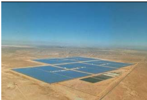
150 MW Parabolic Trough Plant Kramer Junction, CA
