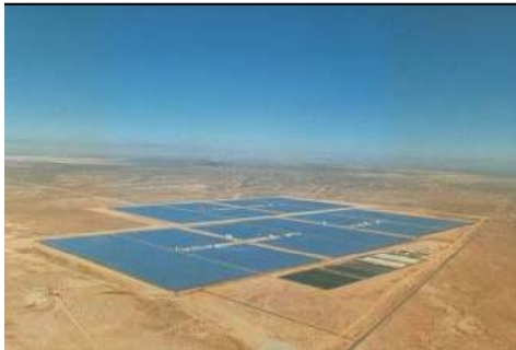
150 MW Parabolic Trough Plant Kramer Junction, CA
