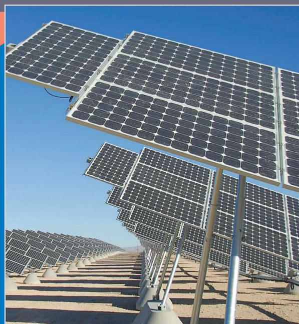
This 14.2-MW PV power plant at Nellis Air Force Base, Nevada, is one of the largest solar power plants in the world using flat-plate PV technology.
