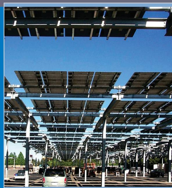
This 540-kilowatt flat-plate PV system installed at the Cal Expo in Sacramento, California, produces enough energy to power about 180 homes and provides shading for some 1,000 vehicles.
