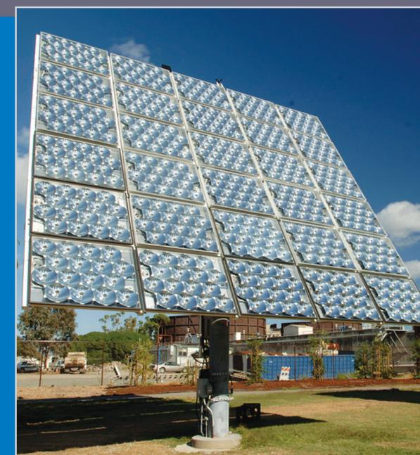
The SolFocus CPV system shown above is mounted on a dual-axis tracker that maintains the alignment of the optics with the sun.
