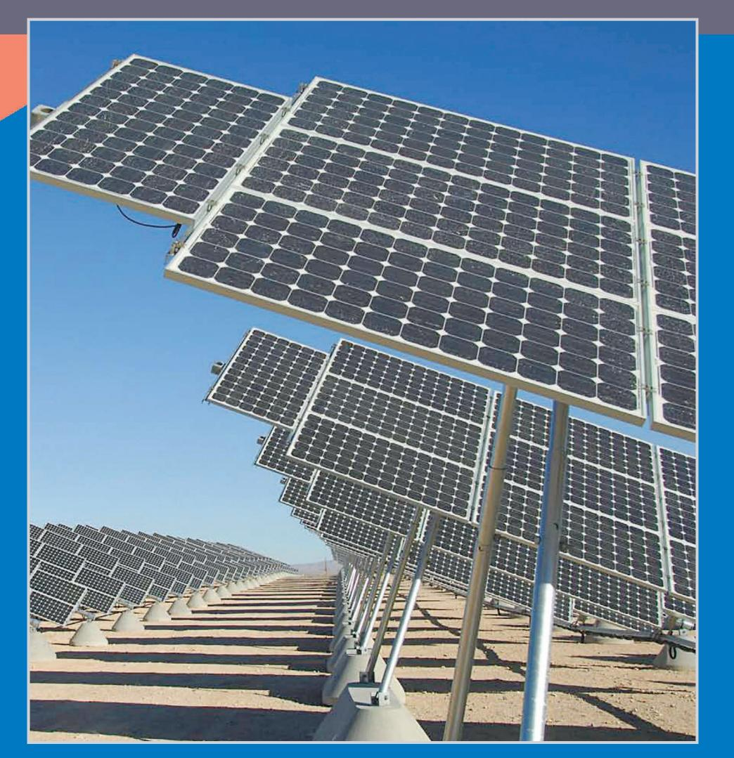
This 14.2-MW PV power plant at Nellis Air Force Base, Nevada, is one of the largest solar power plants in the world using flat-plate PV technology.
