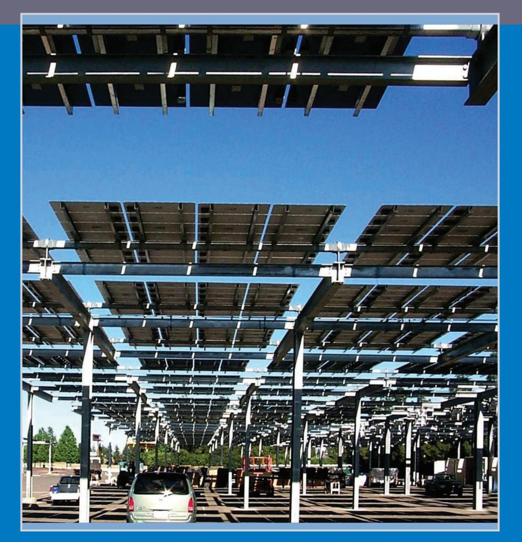
This 540-kilowatt flat-plate PV system installed at the Cal Expo in Sacramento, California, produces enough energy to power about 180 homes and provides shading for some 1,000 vehicles.
